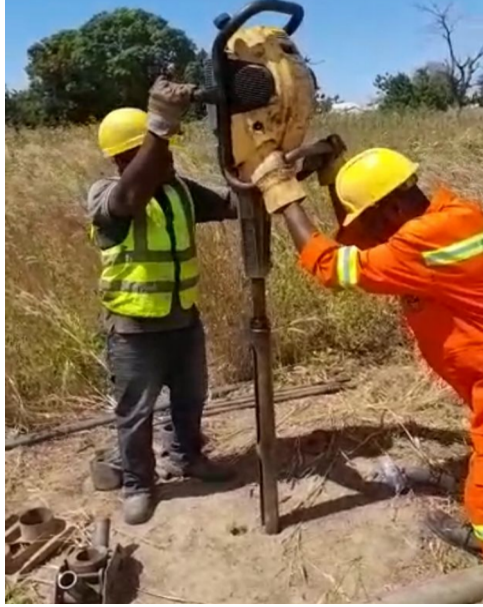
Figure 4: An image of an Auger drill in operation
